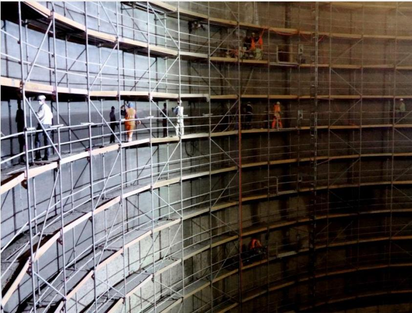
Major damage was detected after a major fire in a sugar silo. There were very large cracks and concrete bursts visible on the surface. As a result, the sugar silo was no longer usable.
