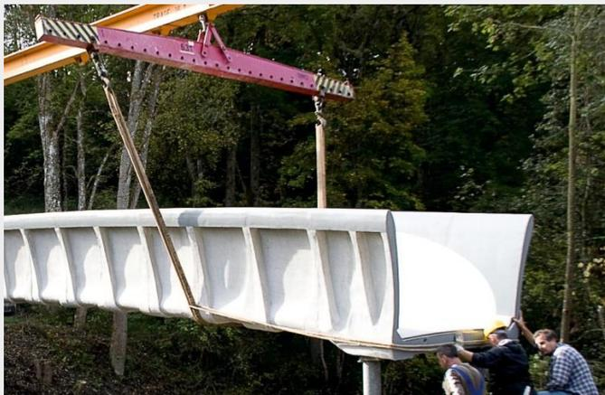
The textile concrete bridge is the second of its type and has double length of its predecessor model in the Saxon city of Oschatz.
