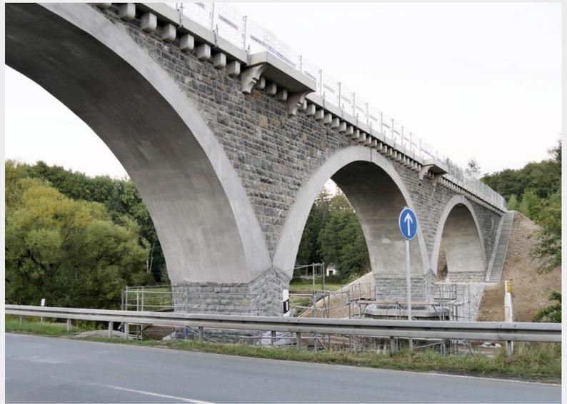
After an elaborate examination of all the available redevelopment techniques, the arches were repaired using carbon reinforced concrete, due to its clear advantages. Two layers of carbon grid were installed and covered using spray concrete lining. The thickness of the carbon concrete was only 20 mm in total, which would not have been remotely possible with steel reinforced concrete.
